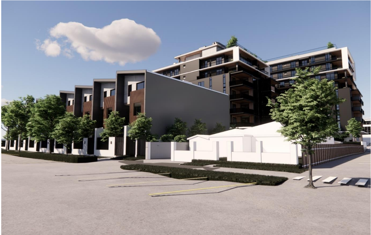
FIGURE 19. ARTIST IMPRESSION OF PROPOSED CIVITAS STAGE 3 – STREET VIEW FROM MURRAY STREET LOOKING AT THE NORTH-EAST CORNER
